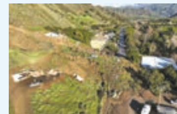
2023 mudslides continue to cripple highway 150.
